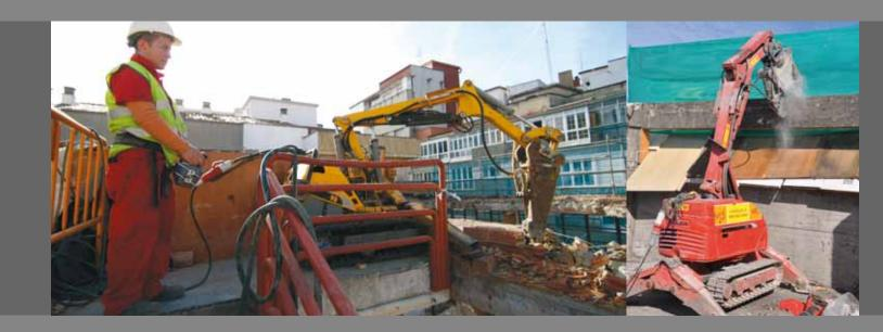
Demolitions using distance controlled robots equipped with hydraulic crushers and hydraulic hammers.
