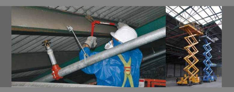
Different works are performed such as removal and dismantling of materials with asbestos, non friable asbestos such as asbestos cement (better known as materials made of slate) and friable such as boiler insulators, projected asbestos, etc.
