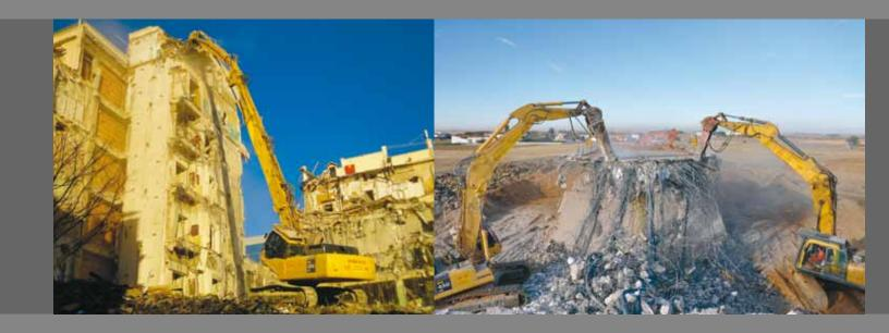
Demolitions in high places are carried out safely, quickly and a correct separation of the materials in the original place is made to maximize the recycling and to minimize the debris volumes that must be transported to the tank.
